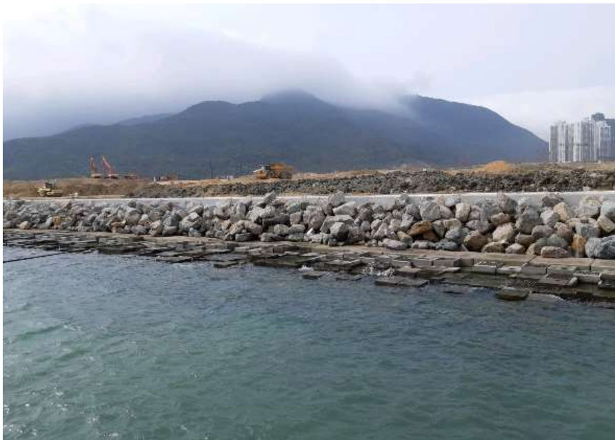
General View of Rocky Eco-shoreline
